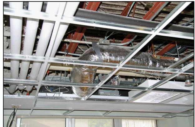
The use of smaller piping in active beam systems also addressed the challenge of extremely low floor-to-floor heights and restricted plenum space by eliminating the need for large ductwork. Humidity was not an issue in the space, as this was readily controlled through the primary air handler, ensuring that only air with the desired moisture level would be delivered into the space. Moisture sensors were incorporated into the Price Active Beams as well.
