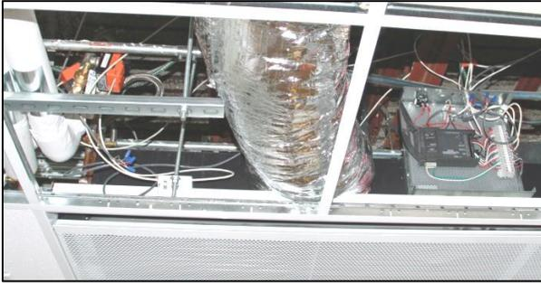
Since the hospital does not run chillers during the winter months, the need for an alternate cooling source became essential. Innovative engineering by BSA incorporated the cooling coils of two existing air handlers in the mechanical room as dry-coolers for the chilled beam system. Ultimately this arrangement provides “free cooling” for CAMC during the winter months.
