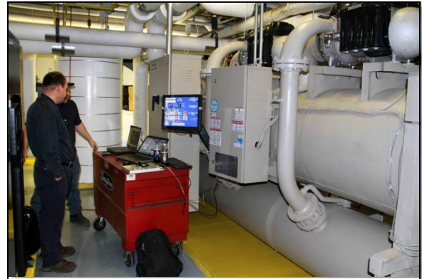
A certified Daikin Technician fine tunes the unit’s controls during installation.
